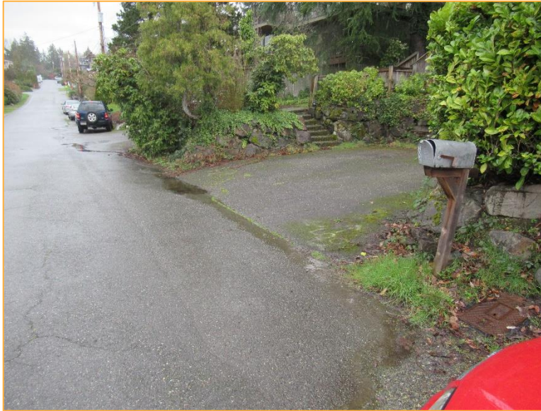
Photo 1 – Facing northwest along the front of the lot, on-site runoff sheet flows into 67 th Ave SE and flows north until discharging into the catch basin beneath the blue Jeep.
