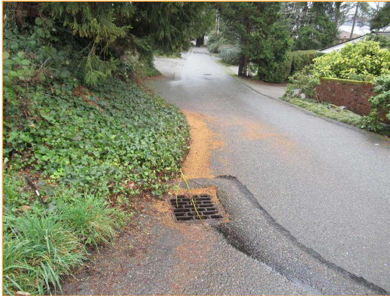
Photo 11 – Facing south at catch basin 18c-144. Stormwater continues south through catch basins 18c-142, 18, 134, 147, 136, and 163 in that order.
