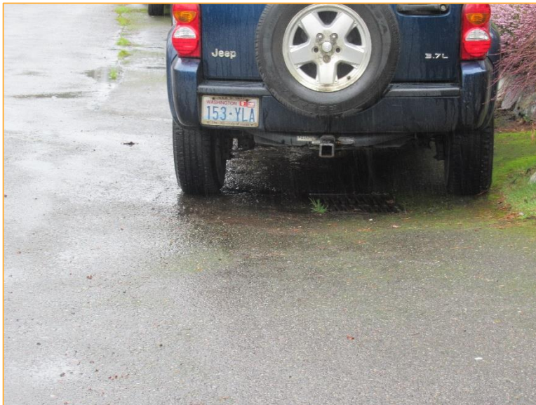
Photo 2 – Facing northwest, stormwater from the site enters this catch basin (18c-26) at the northwestern corner of the property.
